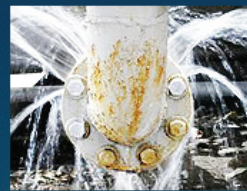
Leaking Pipe 09/12/2012
